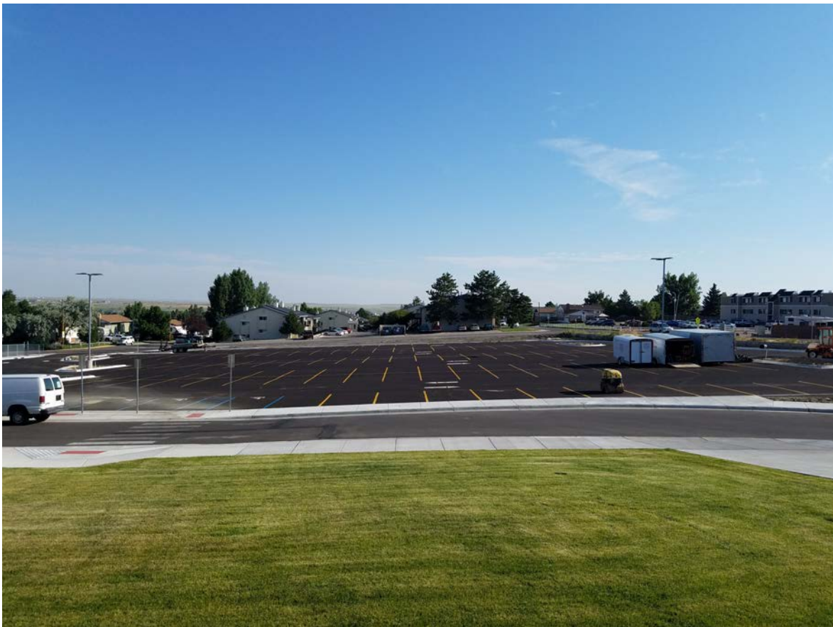
New North parking lot completed, 169 spaces
