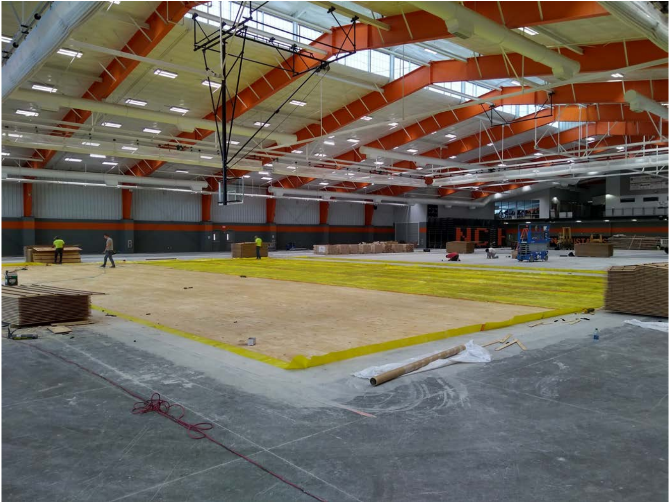
Wood gym floor installation & suspended basketball goals
