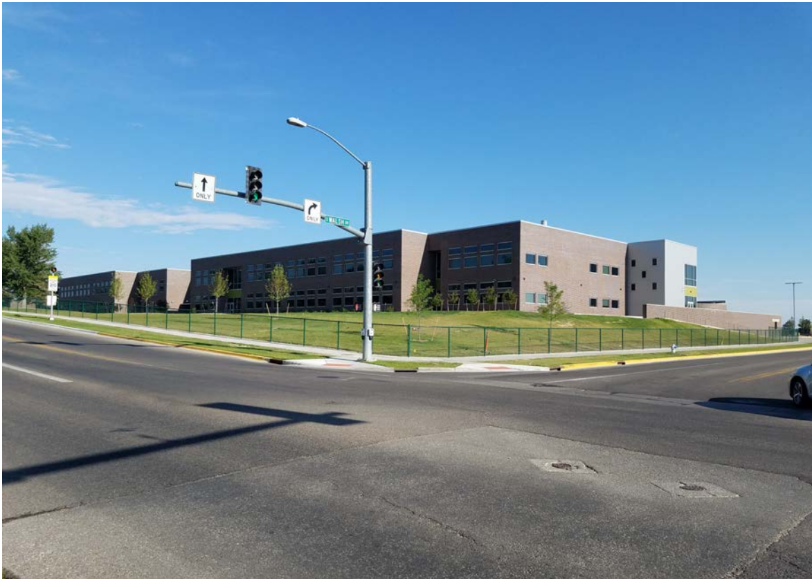
New safety & security fencing along 12 th St & Walsh Dr
