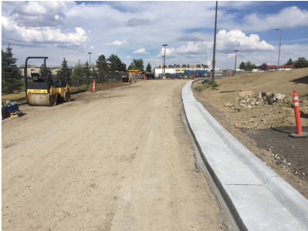
Kelly Walsh Drive Curb and Base – Viewed from South
