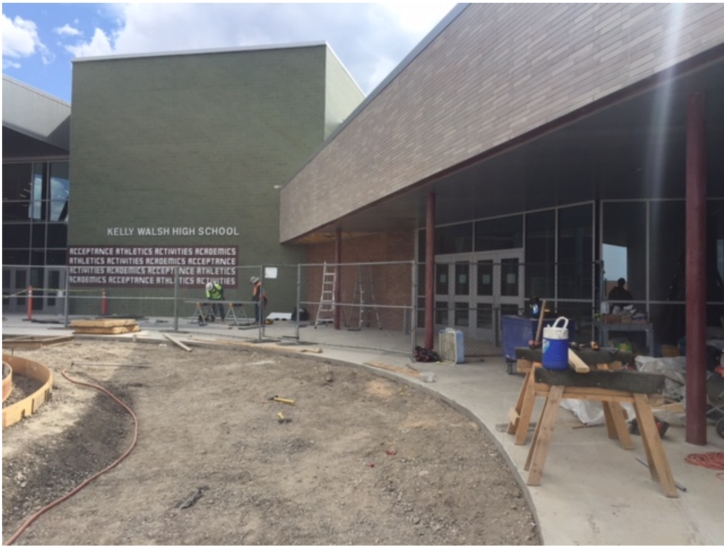
Main Entrance/Music Wing Site Work – Viewed from NW
