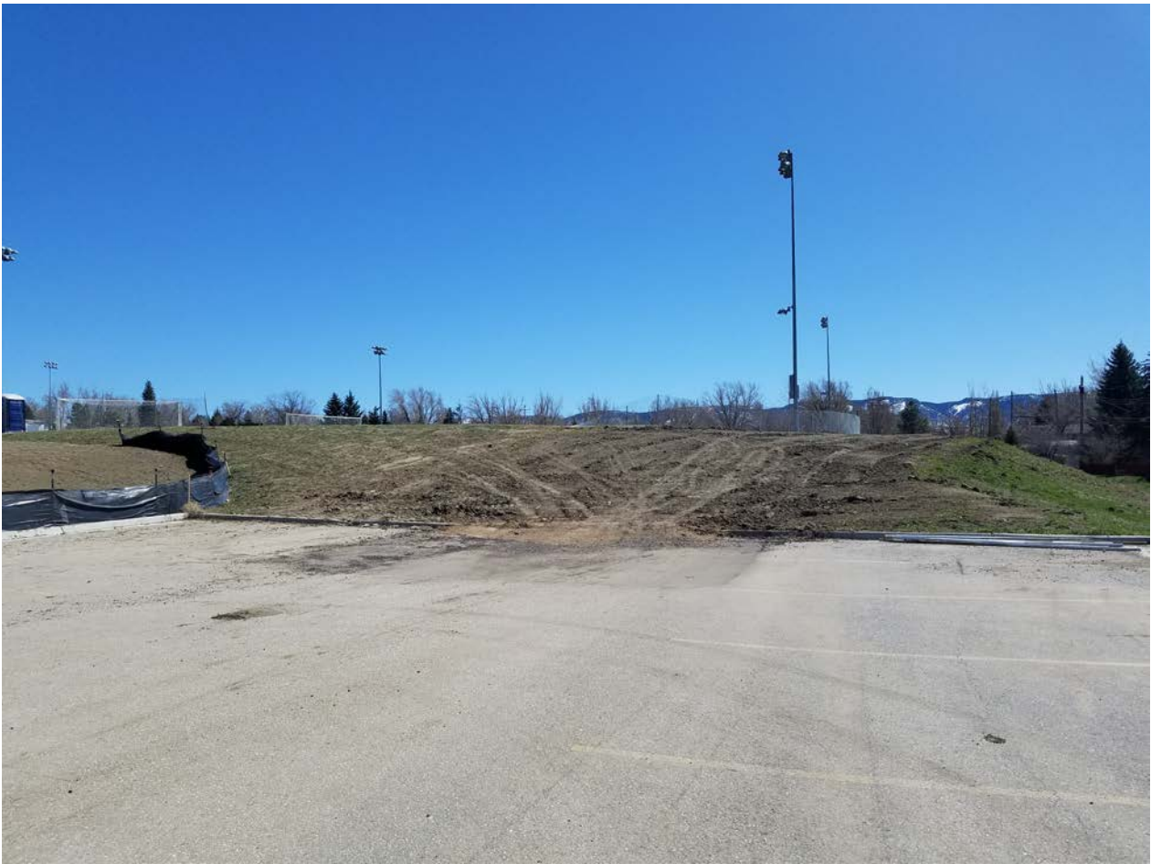
Temporary Road to NW parking lot removed
