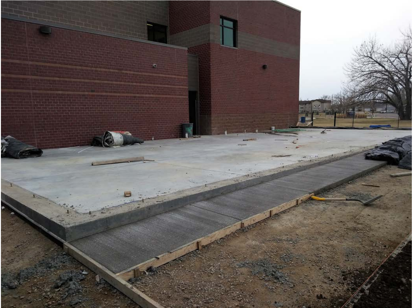
Lincoln Pre-School Classrooms (Floor slab & sidewalk)
