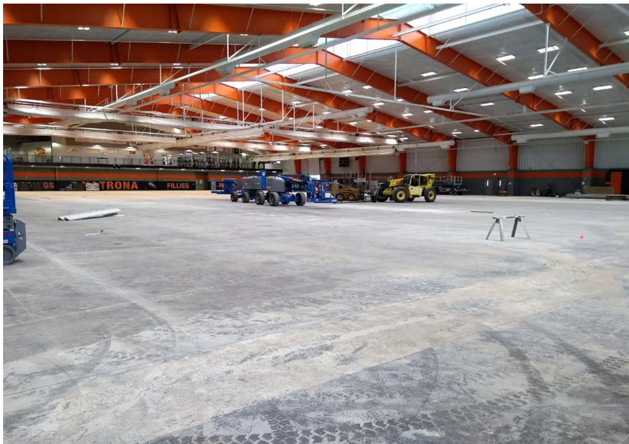
MACC Curtain Framing and layout for depressed slab and track
